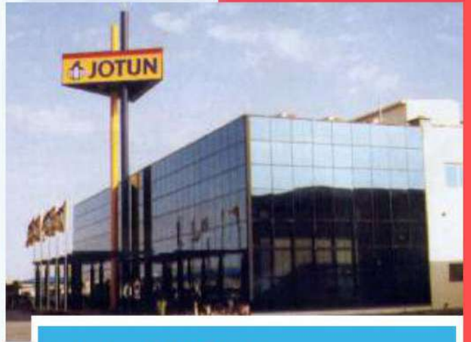
Jotun UAE Ltd Al Quoz-Dubai - Warehouse
